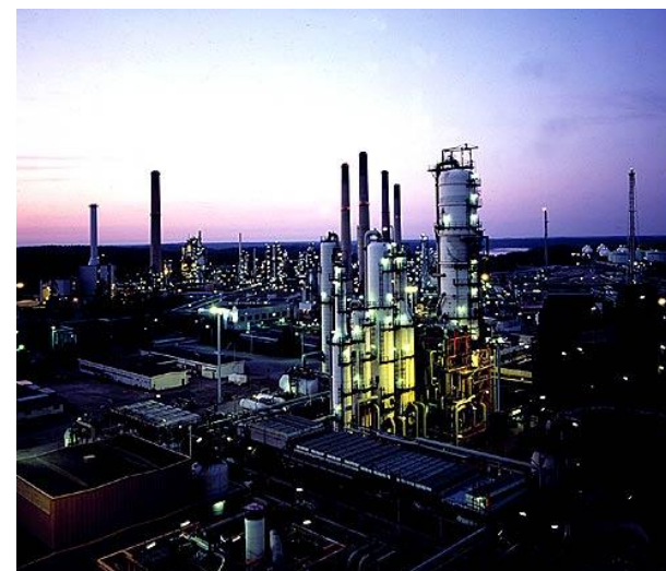
Neste Oil Porvoo Refinery Diesel Project, Porvoo Kilpilahti, Finland
